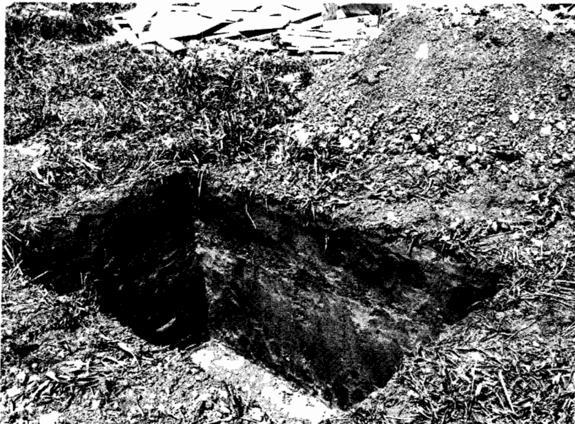
The pit should be in a well-drained spot. It should be 3 1/2 feet deep, 3 1/2 feet wide. Allow six feet in length for every 200 pounds of meat. The dirt should be thrown well back to provide ample work space.
