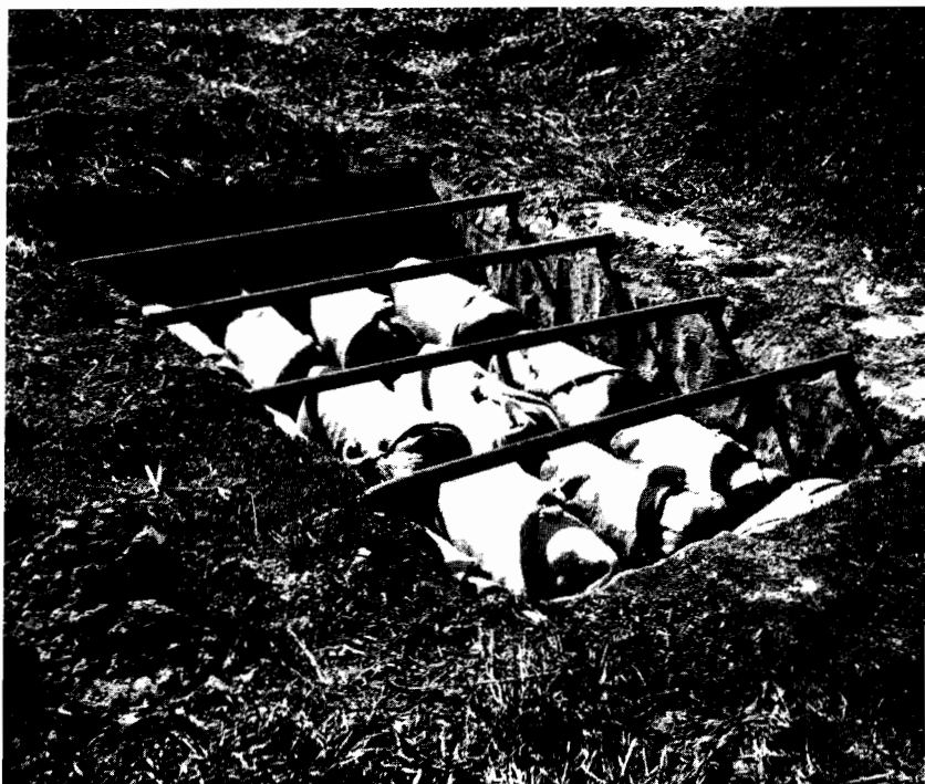
When light metal is used to cover the pit, pipes, rods, or steel fence posts are laid across the trench for added support.
